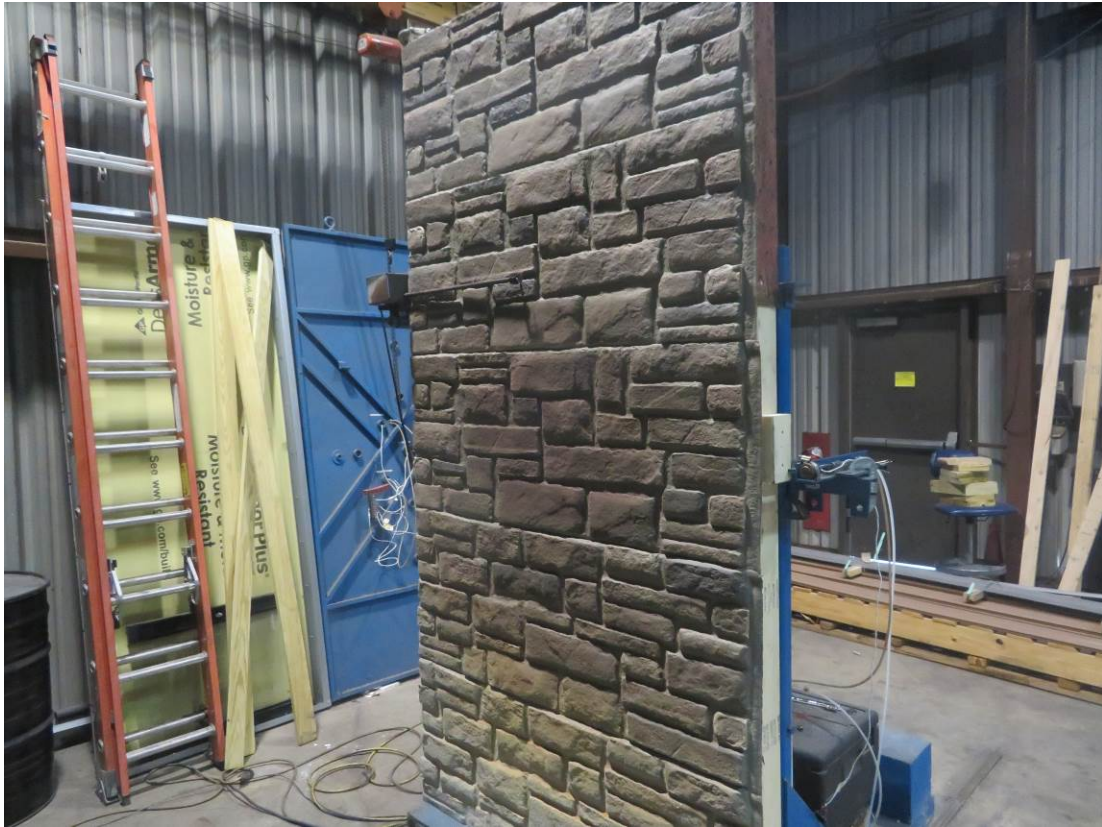
Figure B-3. Sample after fire exposure.
