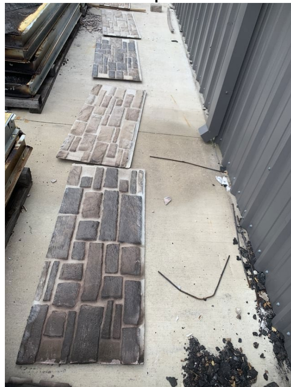
Photo No. 6 Post-Test Exposed Section 2
